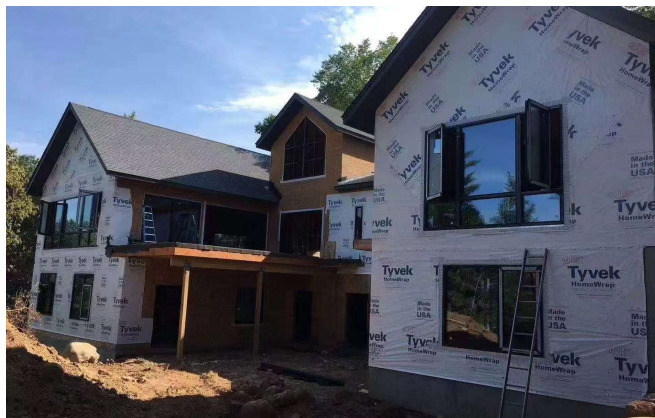
SUPPLIER PROJECT | WINDOW INSTALLATION
